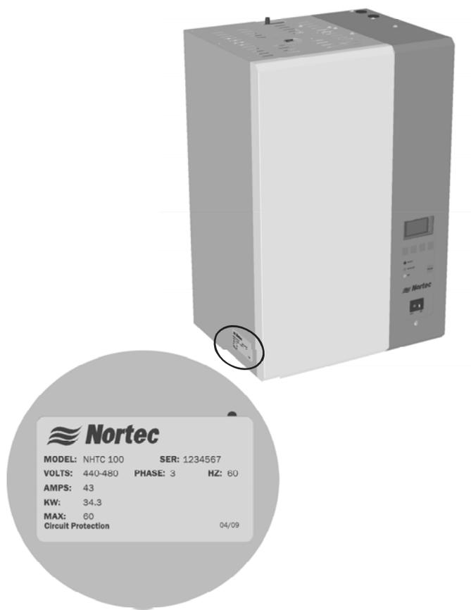
Figure 1: Specification Label Location
