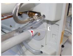
Fig. 49: Install pump
