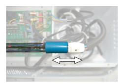
Fig. 74: Remove connection cable
