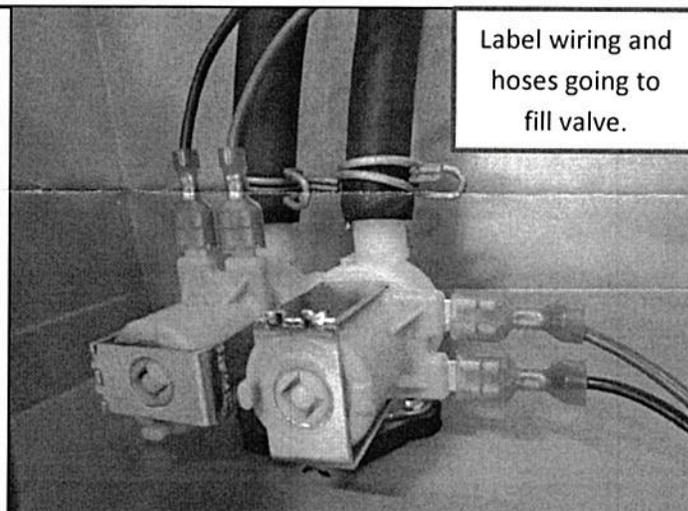
Label wiring and hoses going to fill valve.
